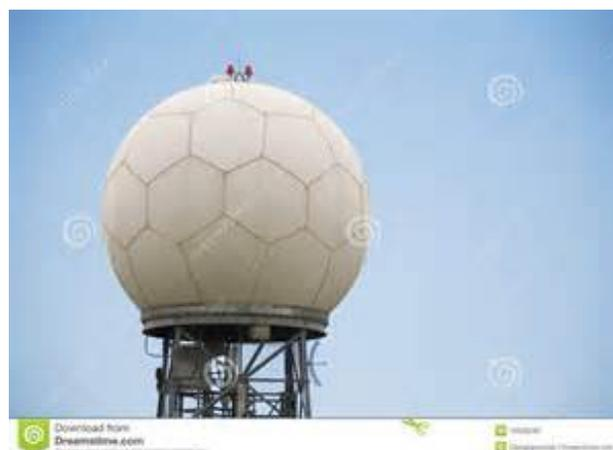
**Figure 4-6 Doppler radar dome**
