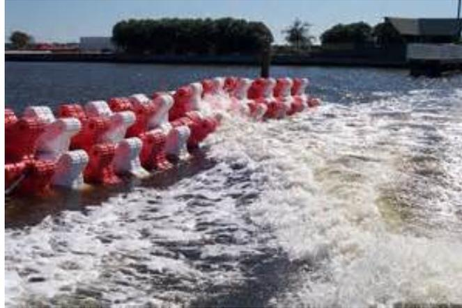
**Figure 4-3 Floating wave attenuator system**
