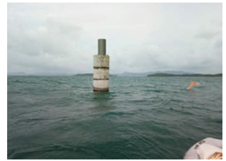
Fig.5 Preliminary construction at sea.
